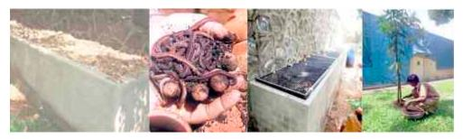
**Use of Organic Wastes Converter** @ **L-Center ,Banglore -** The Organic waste Converter was installed to to convert food waste into bio-fertilizer/manure. This manure is used within the campus for landscaping.
