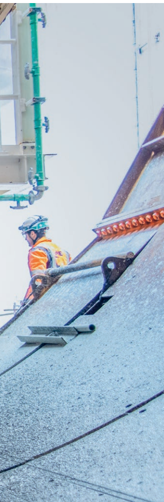
Image: Men at work in the Grand Paris Express construction site.
