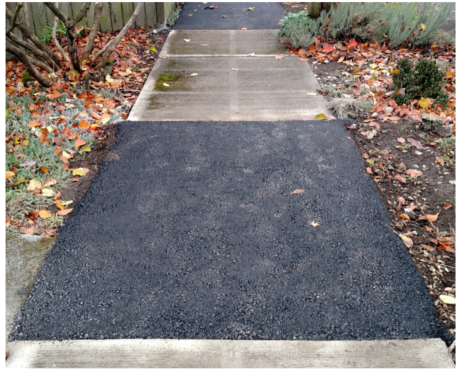
Asphalt sidewalk repair on Charles St
