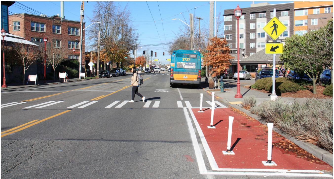
Low cost measures reduce pedestrian crossing distances on Beacon Ave S.
