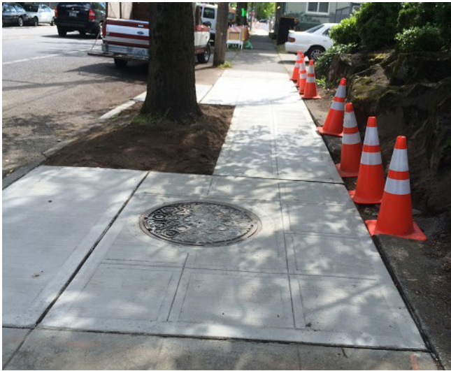
Concrete sidewalk repair on E Cherry.
