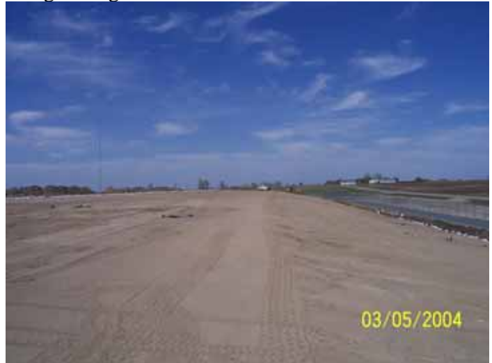
Sand drainage layer placement at Clay County Landfill.
