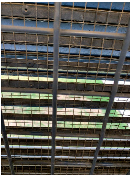
Figure 13: Close up of MITA HCA, grille covering the windows.
