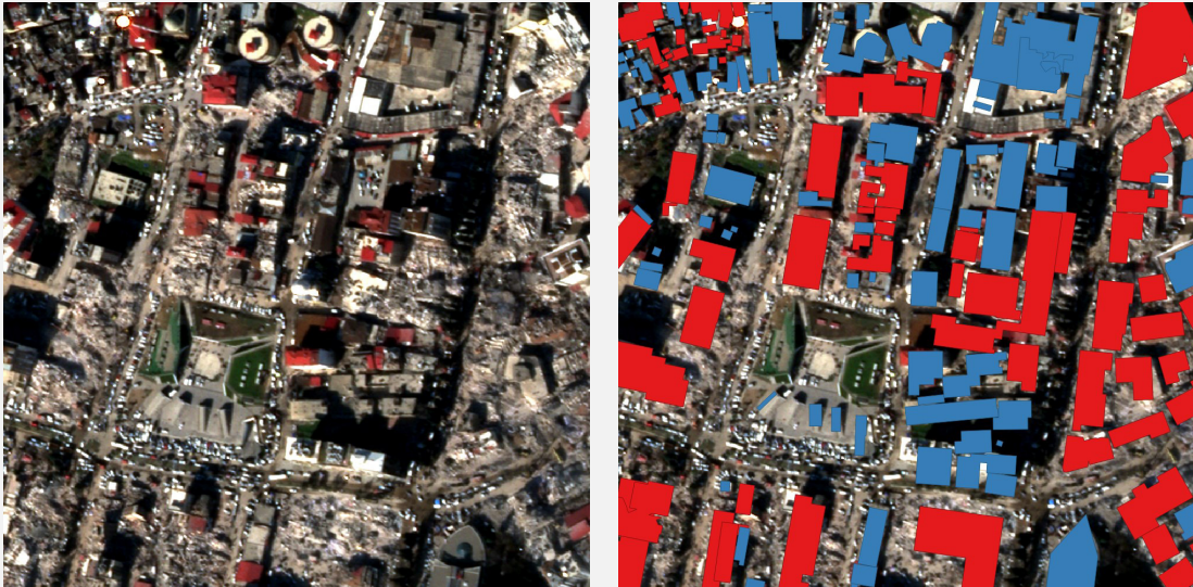
Figure 4: Extensive damage around the Culture Park area of Marash. Planet Labs PBC, February 9th.
