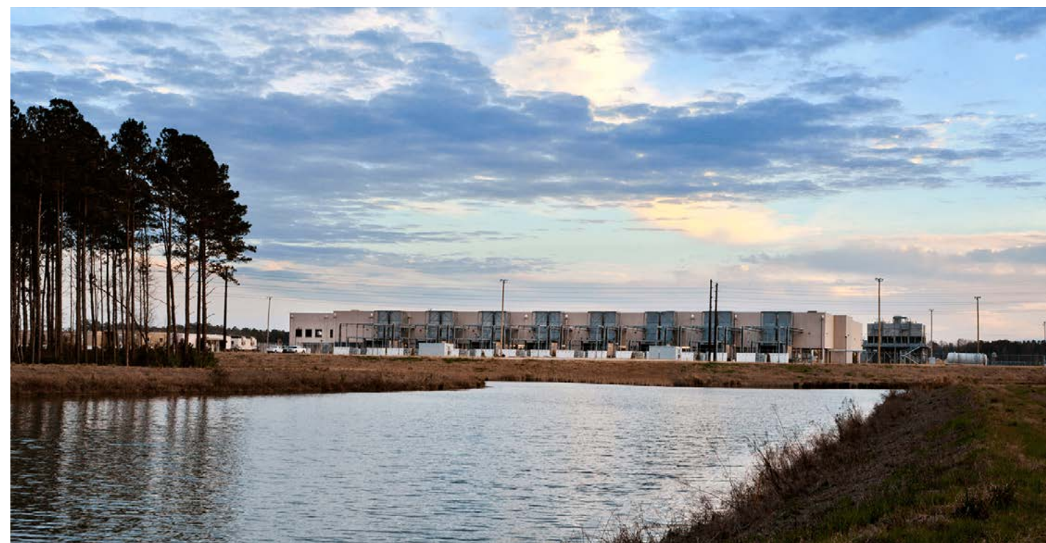
A rainwater retention pond outside our data center in Berkeley County, South Carolina.
