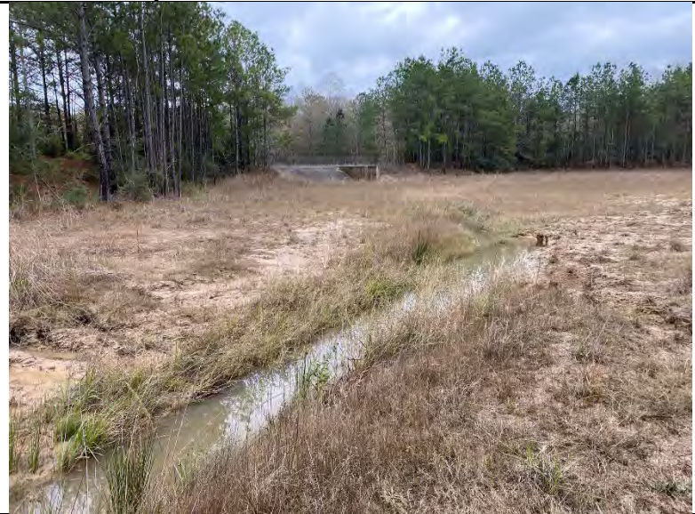
Photo IMG-2041, view of Ditch 2.
