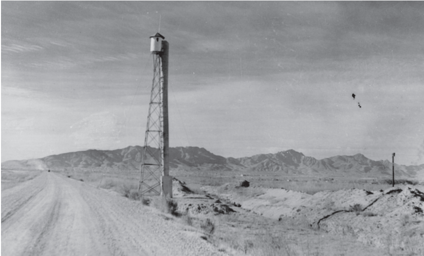
Border patrol, 65 foot steel tower used by U. S. Border patrol for watching Rio Grande River, lead to top is enclosed so no one knows when a border patrolman enters. Tower built by WPA.
