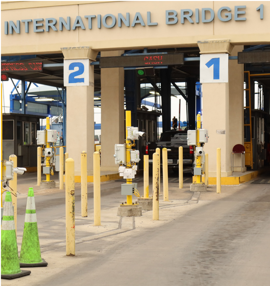
Automated License Plate Readers at the Eagle Pass International Bridge. Source: EFF.
