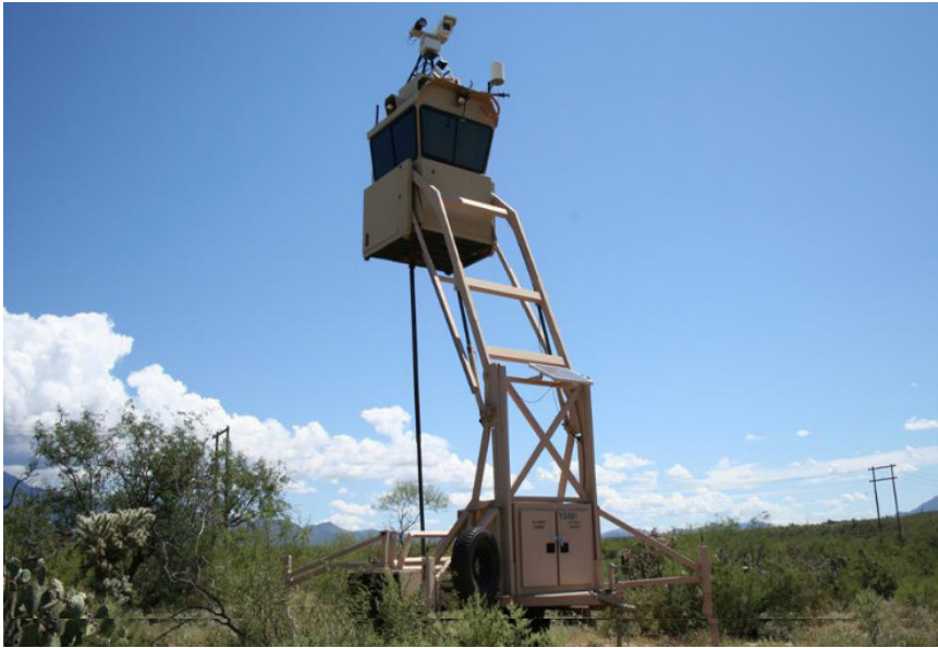
A Teledyne FLIR SkyWatch tower. Source: CBP.
