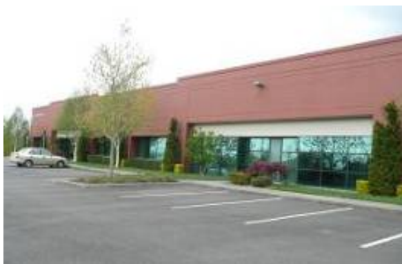
Dedicated office building for testing enterprise WLAN
