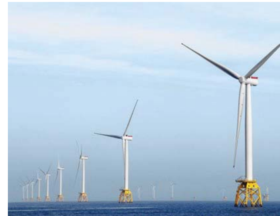
Offshore wind turbines in the North Sea.
