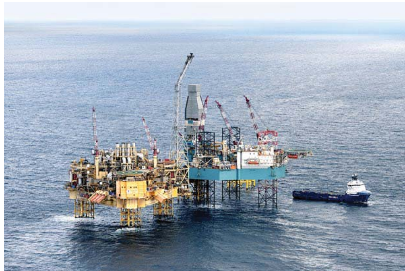
The Elgin-Franklin Platform in the North Sea.
