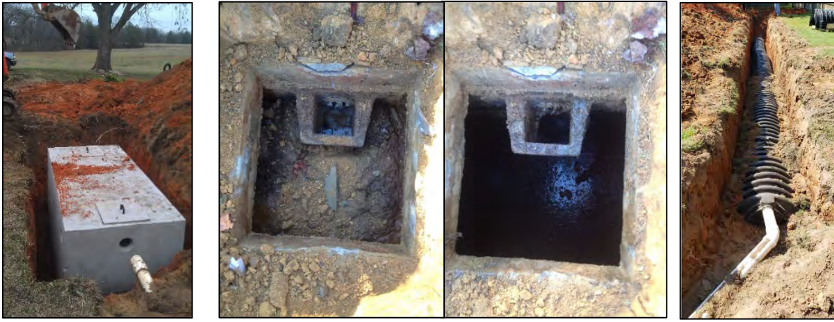
Examples of a Septic Tank Replacement, Before and After Maintenance, and Drainline
