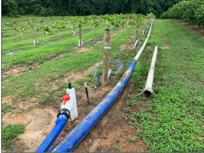
Example of a drip irrigation system installed on muscadine vines
