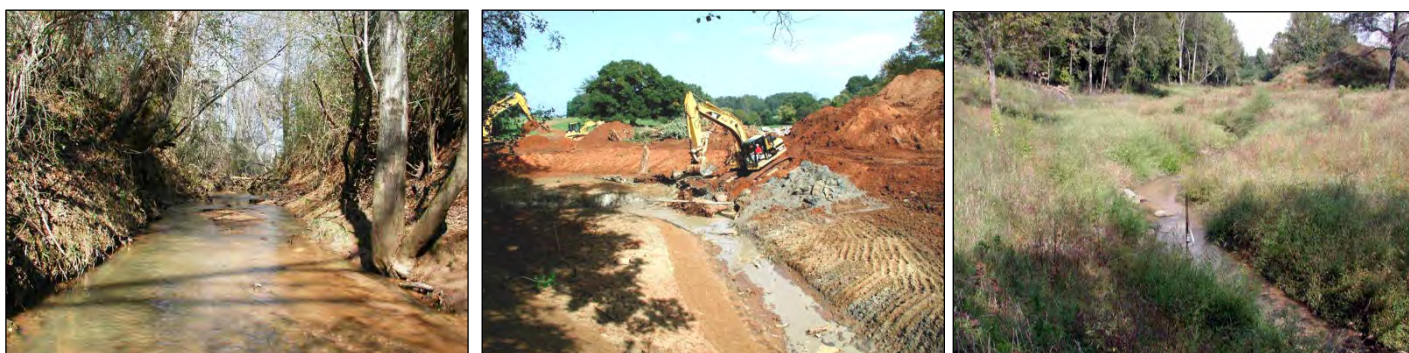
Example of a Riparian Buffer Restoration in Hunnicutt Creek, Clemson University – Channelized Stream Overrun With Invasive Species,, During Construction, After Restoration (Source: Clemson University)
