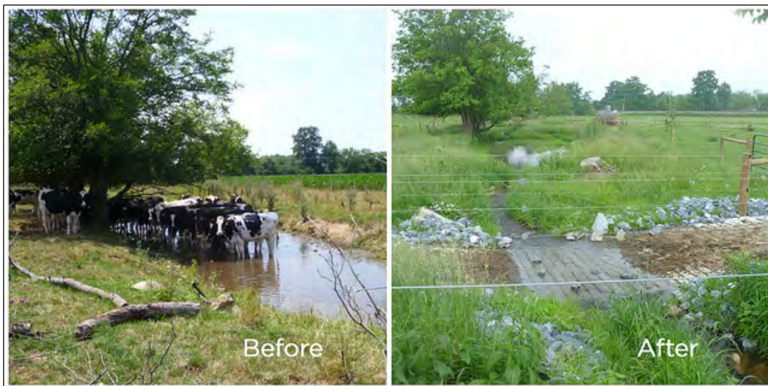
Example of Armored Streambank Crossing (Source: USDA NRCS) 76
