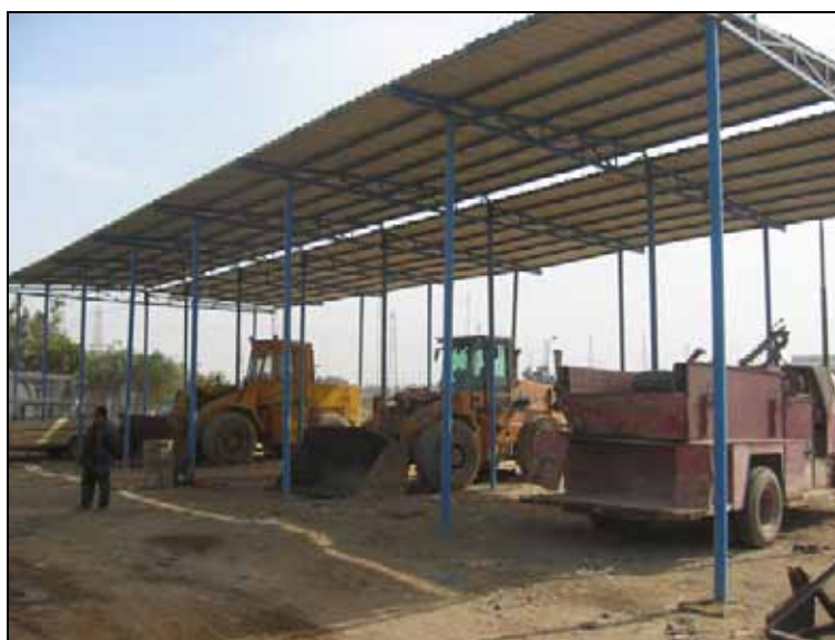
Operational Equipment: Calyobeya Governorate
