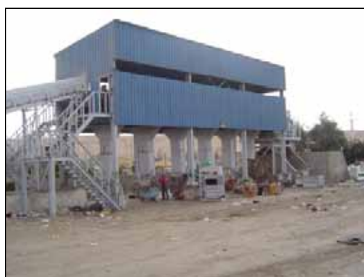
Composting Plant: Cairo Governorate
