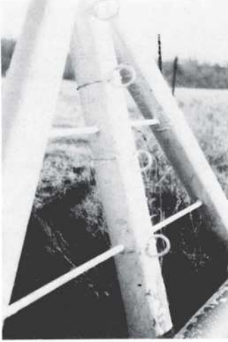
A cattle-guard wing with rings to hold barbed wire, Greenwood County, Kansas
