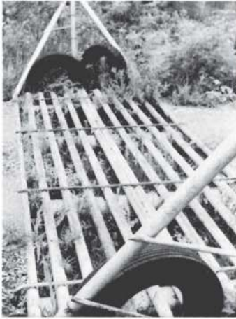
A cattle guard near Virgil, Kansas, built by Mick Sage. Tires were added to help deter livestock.
