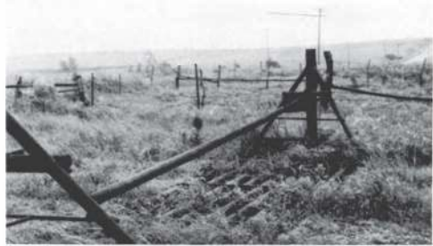
A cattle guard with pipe-bar gate to keep out unwanted automobile traffic, Greenwood County, Kansas
