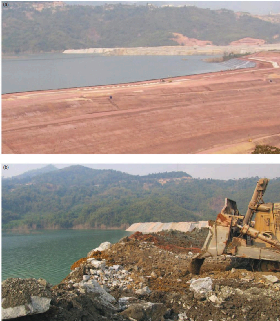
Figure 15.3: (a) Waste rock deposition in the tailings storage facility, (b) pushing waste rock lifts into the tailing pond. Source: W Wilson
