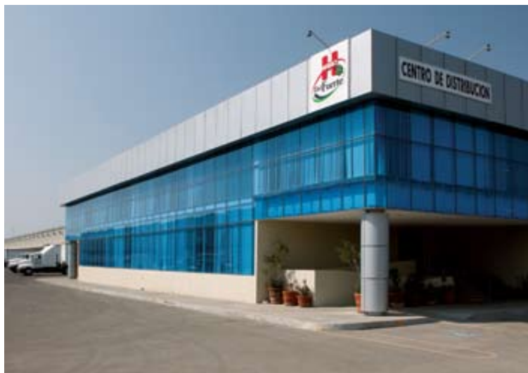
“El Convento” New Distribution Center located in the State of Mexico
