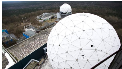
Former US listening station at Teufelsberg, Berlin.
