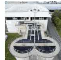
Source: Laing O'Rourke
