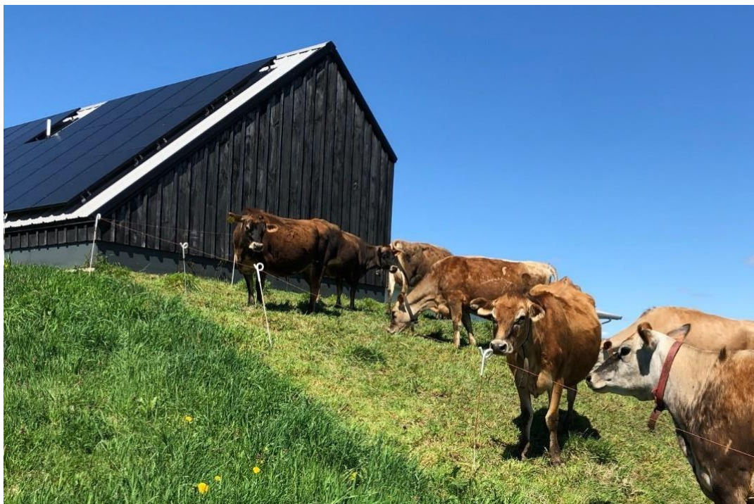
Figure 1: Rooftop Solar array at Sweet & Salty Farm, Little Compton, RI RIAgEP, REAP, and the Renewable Energy Fund were all used to fund this project
