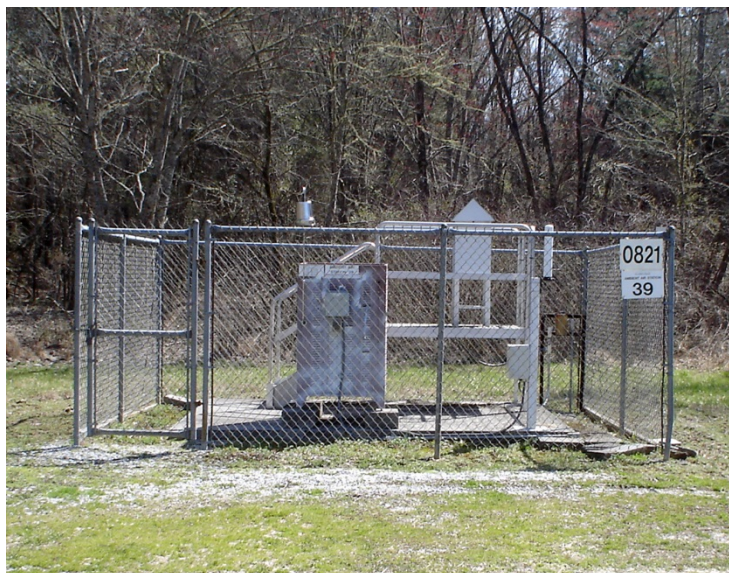
Fig. 6.3. Oak Ridge Reservation ambient air station.
