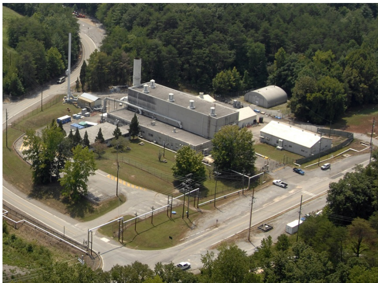
Fig. 5.40. The Molten Salt Reactor Experiment facility.
