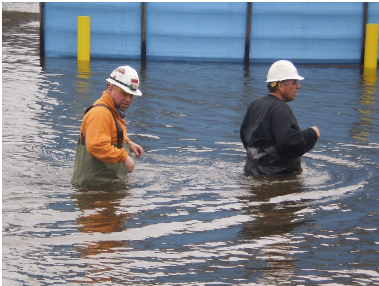
Figure 19: Veolia Water's Mike Ponte and Teddy Demarco wading through flood waters as they go about the unusual business of dealing with historic flooding at the Cranston wastewater treatment facility just outside the flooded maintenance building on March 31st, 2010. (Veolia Water)
