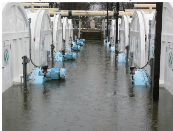
Figure 21: Bristol's Rotating Biological Contactors going under water as local flooding throughout the town makes its way to the treatment plant on March 30th, 2010. (Bristol)
