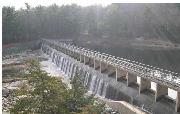
Figure 2: The Gainer Dam spillway on a normal day, with only a trickle being added to normal flows that come from the dam's central outlet, which feeds the North Branch of the Pawtuxet River. See Figure 3 for an image of the spillway's raging torrent on March 31 st , 2010 (NWS/NERFC)
