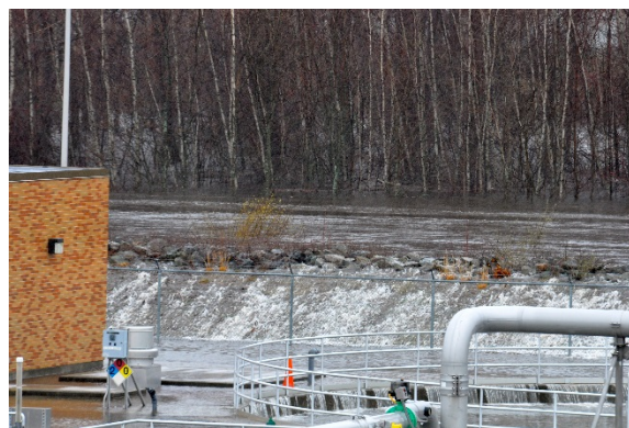
Figure 13: Warwick's 18-foot levee overtopped, bringing water into the plant and flooding process tanks and buildings soon after. (WSA)
