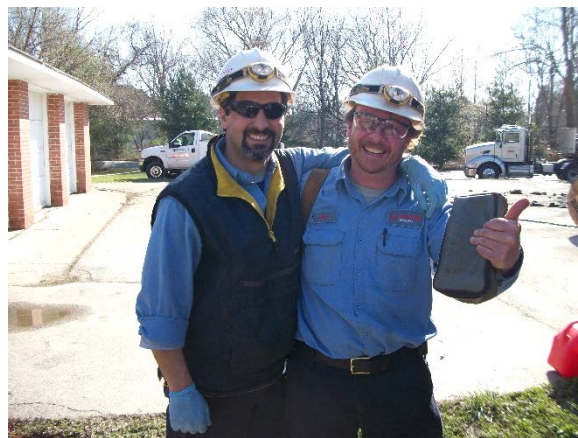
Figure 25: With the waters receded and the sun returned, Veolia Water’s Jack Branco (left) and Jay Keefe celebrate after long hours of powering up the flooded, bypassed Pontiac Avenue pumping station in Cranston.
