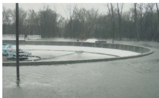
Figure 6: The Pawtuxet River rises towards the five-foot flood protection walls of West Warwick’s secondary clarifiers on Tuesday, March 30th as plant staff evacuate. (West Warwick)
