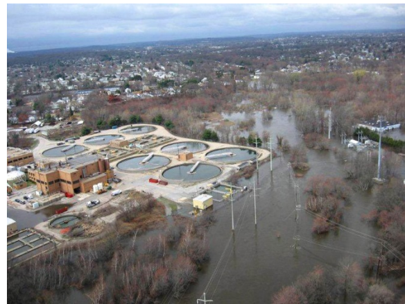
Figure 18: The Cranston wastewater treatment facility after the Pawtuxet had begun to subside. (State of Rhode Island)
