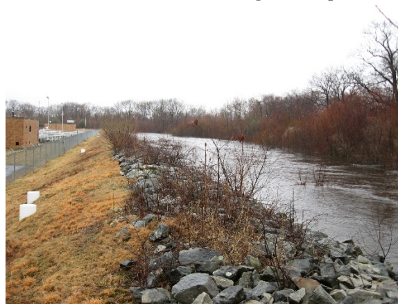
Figure 12: At 14.7 feet, the Pawtuxet threatens but does not overwhelm the 18-foot levee at the Warwick wastewater facility on March 15th. (WSA)
