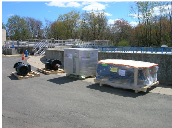
Figure 24: On April 20th, 2010, new equipment arrives at the West Warwick Regional Wastewater Treatment Facility—as water-absorbing foliage appears around the plant—heralding the start of the long rehabilitation of plant equipment. (RIDEM)
