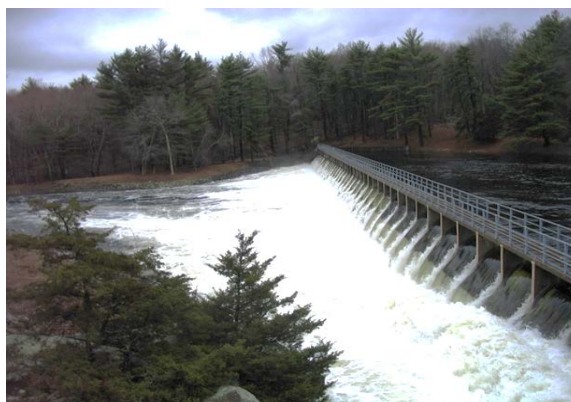
Figure 3: The Gainer Dam spillway at the Scituate Reservoir at 10:30 a.m., March 31st, 2010. Flow was an unprecedented 2.5 feet over the flashboards at a pool elevation of 287.80 feet. See Figure 3 for the spillway on a normal day, with only a trickle flowing over the flashboards. (David Vallee, NWS/NERFC)
