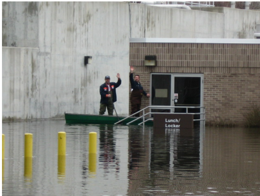
Figure 1: Operators at the flooded West Warwick Regional Wastewater Treatment Facility greet colleagues as they use a boat to assess plant damage after the historic March 30-31, 2010 flooding of the Pawtuxet River.
