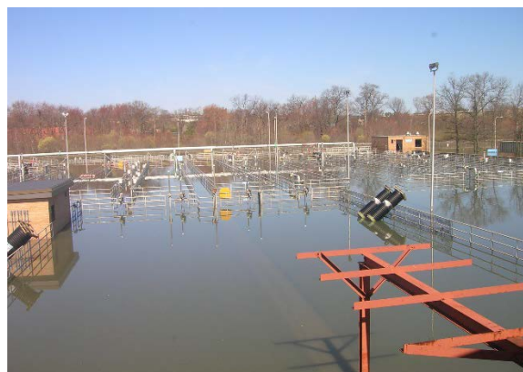
Figure 16: Warwick's wastewater facility on Saturday, April 3rd as flood water continued to be pumped back over the berm. (RIDEM)
