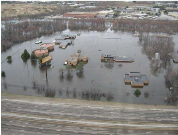
Figure 14: The flooded Warwick wastewater facility sits between the surging Pawtuxet and the closed Interstate 95 on Wednesday, March 31st. (State of Rhode Island)
