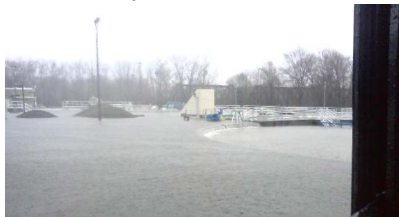
Figure 7: West Warwick's five-foot high secondary clarifiers are overtopped by the rising Pawtuxet on Tuesday afternoon, March 30th. (West Warwick)
