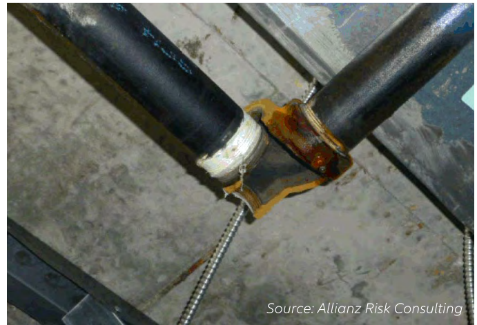
Fractured pipe fitting
