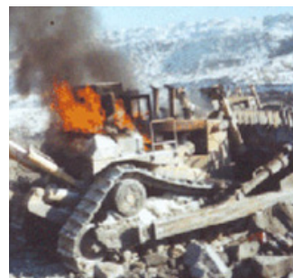
Bulldozer on fire
