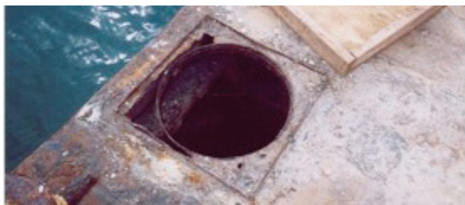
Manhole covered with wooden hatch.
