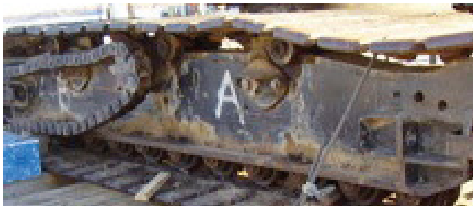
Insufficient securing. Only one (1) \frac{3}{4} " wire looped over treads at each end. Crane mats are not secured to the deck.
