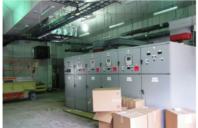
When hot-testing equipment, always have a written commissioning plan
