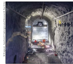
The excavated DUNE cavern.
