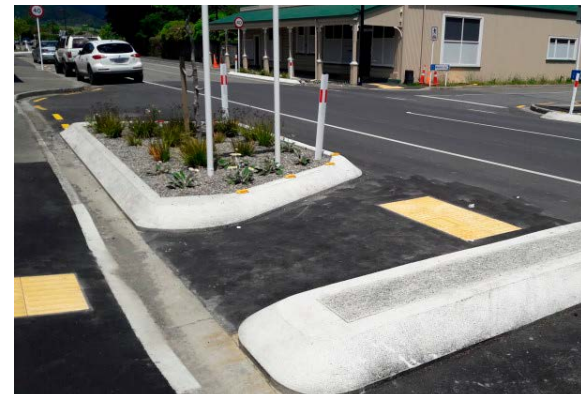
Source: New Zealand Transport Agency (© J Ward).
