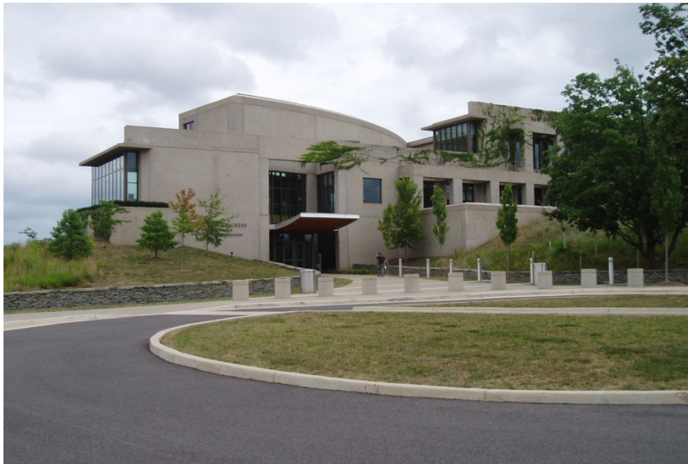
Main entrance to the Library of Congress’ Packard Campus
