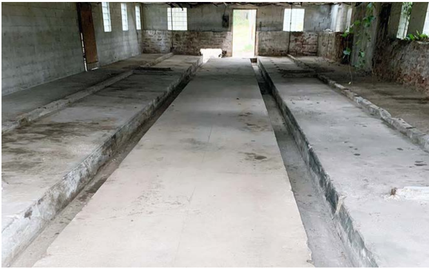
The photos above are from a property in central Wisconsin whose occupants were accepting TVs and other electronics for free. After several years, contractors made progress on a cleanup in 2021.
